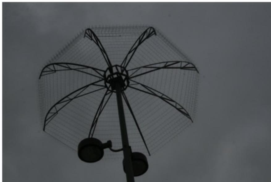
**DAS Pole-Mounted Hemisphere Used to Protect Aircraft Parking Ramp**
